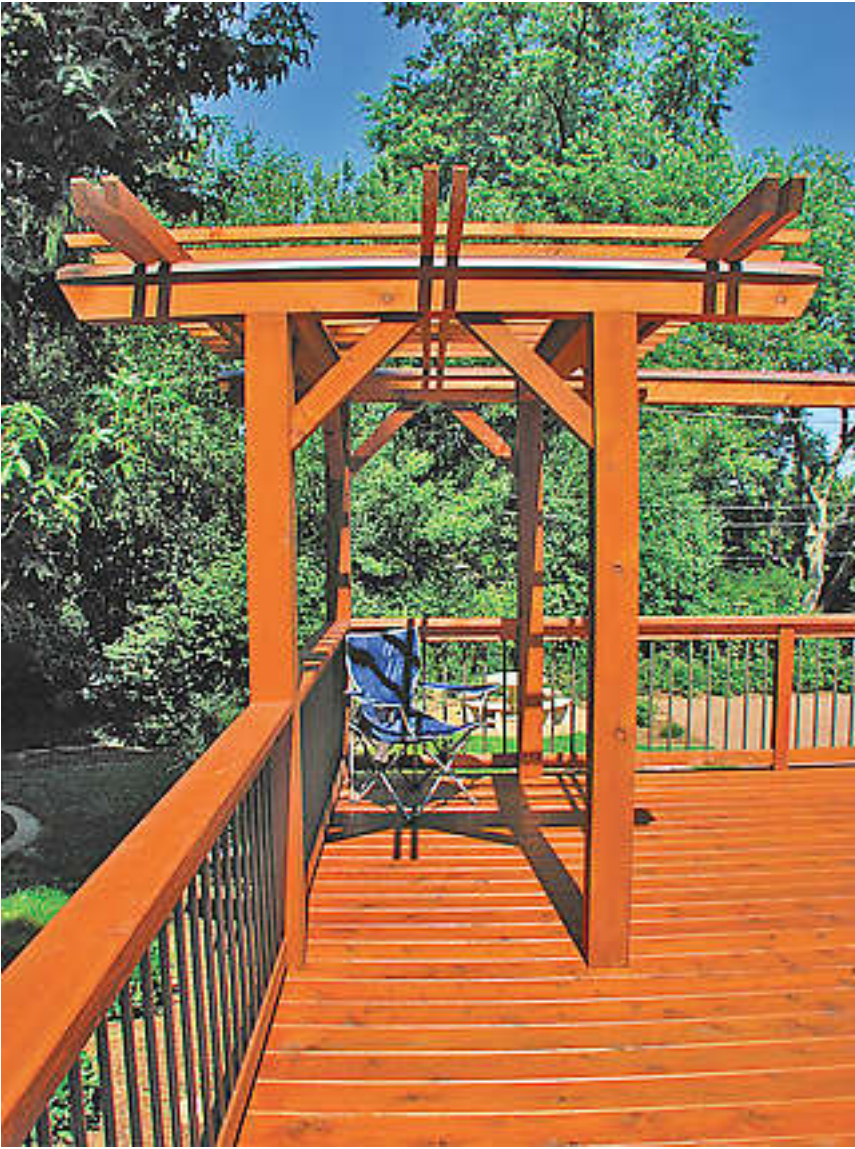
The deck was built with stained western red cedar. Photos by Carrol Krause
